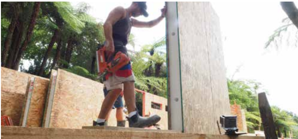
6 Standing the panels. The Formance walls simply slot onto subplate
