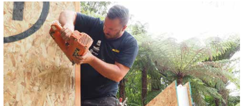
7 Garrick nailing off the timber spline connector ready for the next panel
