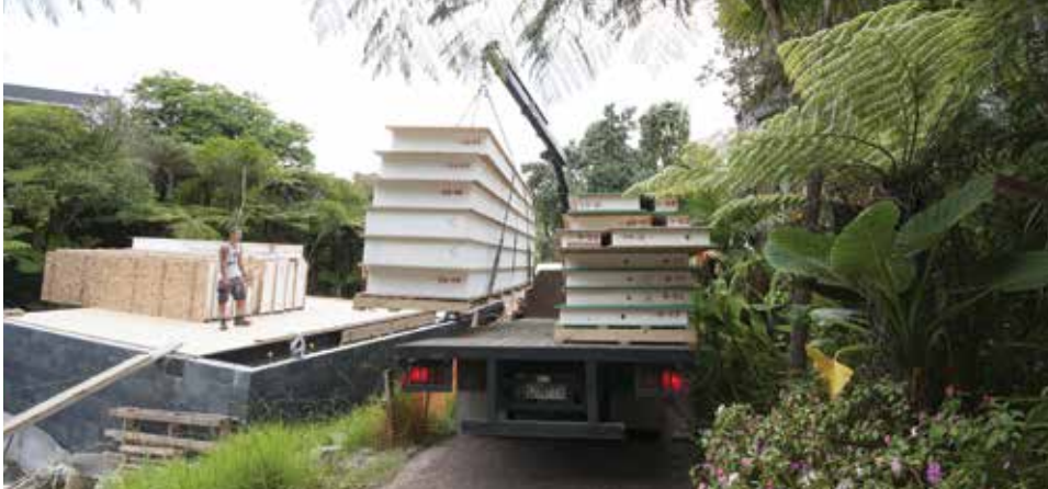
3 Formance Structural Insulated Panels arriving on site
